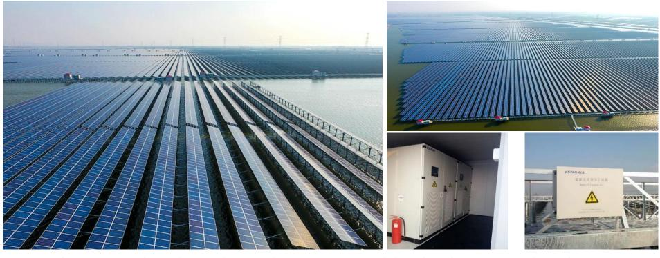
One PV plant is 200MW located in Ningbo City, Zhejiang Province, and the other plant is 150MW located in Jiaxing City, Zhejiang Province. These two PV plants have both been successfully achieved Grid-tied Power Generation since June 2016. KSTAR provided total of 560 units GSL0630 central inverter for this 350MW project(Purchase contract as attached).
